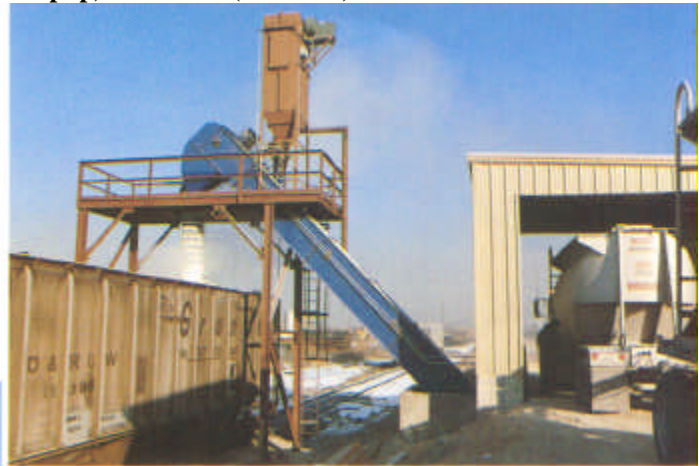
Soda Ash – Unloading 80,000 lb. (trailer & pup) in 20 min. (120 TPH)
