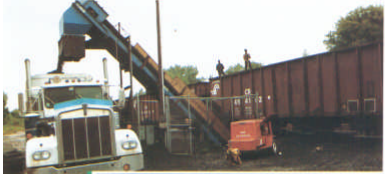
Boiler Coal – Loading a 24 Ton Trailer in 4 minutes (360 TPH).
